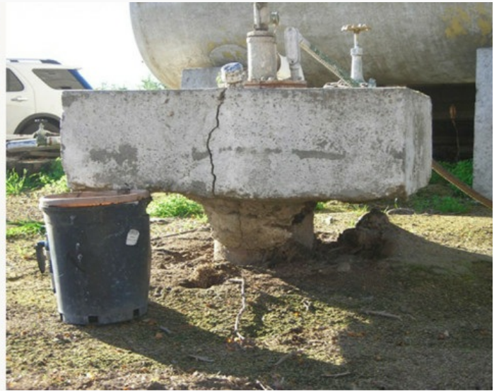
The wall of a canal (left) cracks as the earth around it sinks. The top of a well (right) is pushed up and out of the ground as the ground around it sinks. Credit: U.S. Geological Survey
