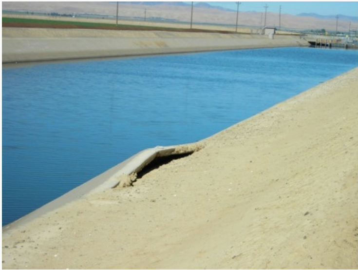
The wall of a canal (left) cracks as the earth around it sinks. The top of a well (right) is pushed up and out of the ground as the ground around it sinks. Credit: U.S. Geological Survey
