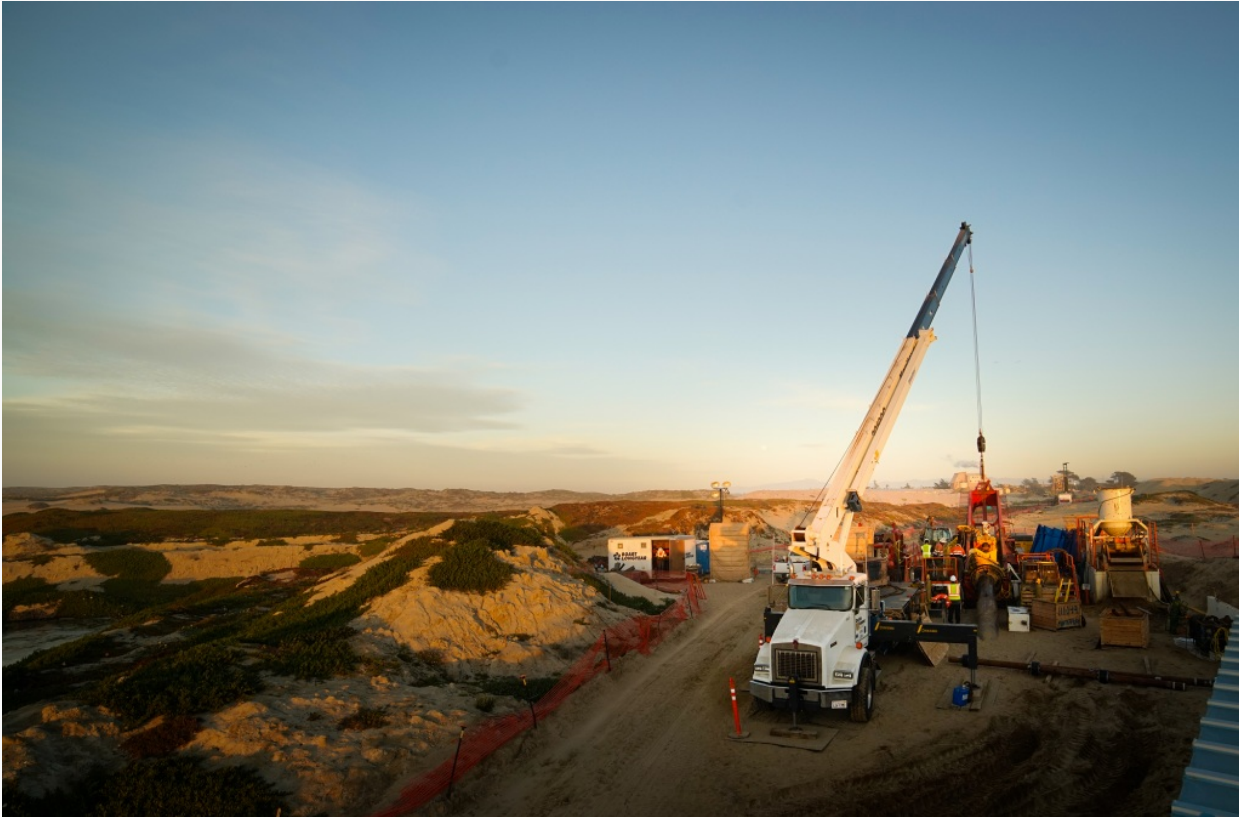
The California American Water Company plans to desalinate water from Monterey Bay. This drill site near the town of Marina is meant to prove they can access seawater from under the beach. (Luke Gianni/California American Water Co.)
