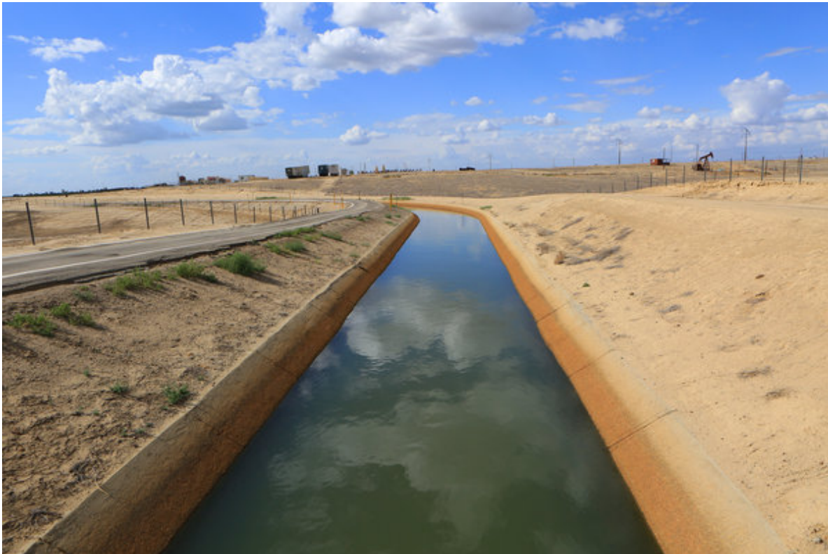
Water from the oil field is cleaned and released to a local water district, which sells it to agricultural buyers for irrigation. Credit Jim Wilson/The New York Times
