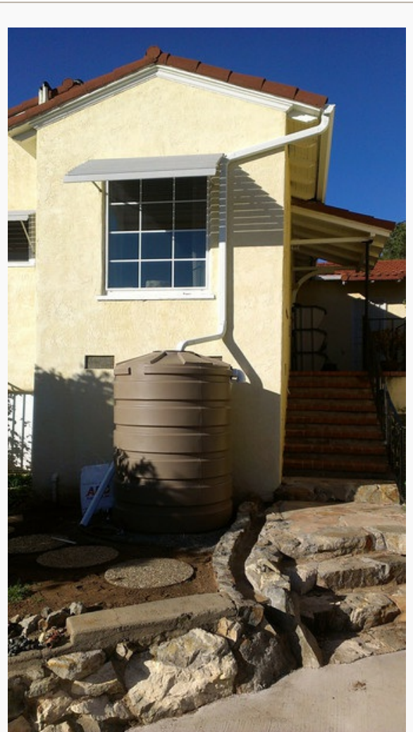
Many Australian homes now have rainwater capture systems. (Albert Barlow, Rain Water Systems)
