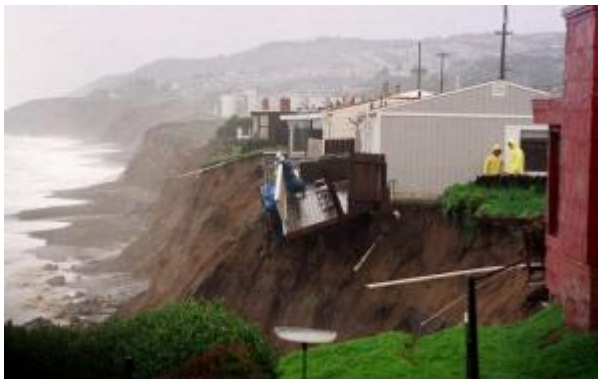
The deck of a Pacifica home hangs precariously over an eroding bluff in February 2008, during a winter of heavy storms. (Associated Press)
