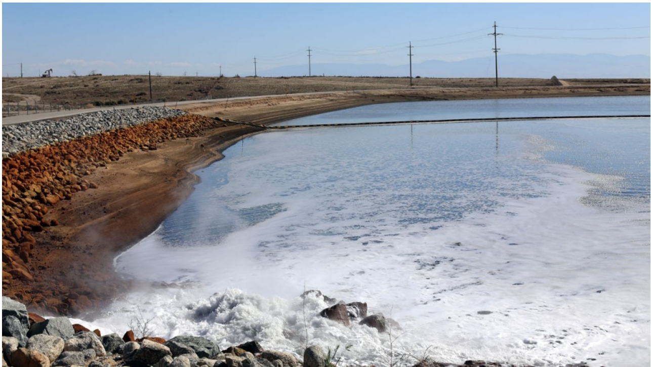
Water from Chevron gushes out of a pipeline in a reservoir that serves the Cawelo Water District. (Lauren Sommer/KQED)
